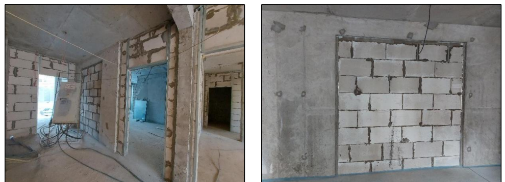
Figure 4. General design solutions for non-load-bearing structures.
