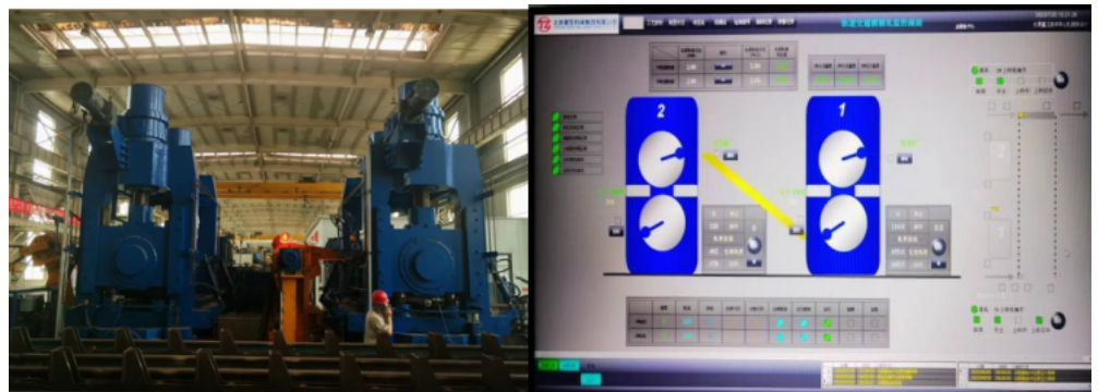
Figure 13. Intelligent control platform for rolling mill site.
