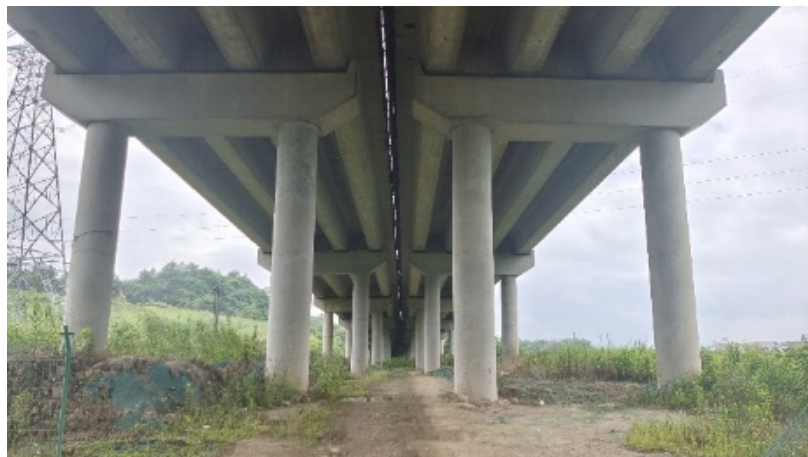
Figure 8. Huangshan River Bridge.
