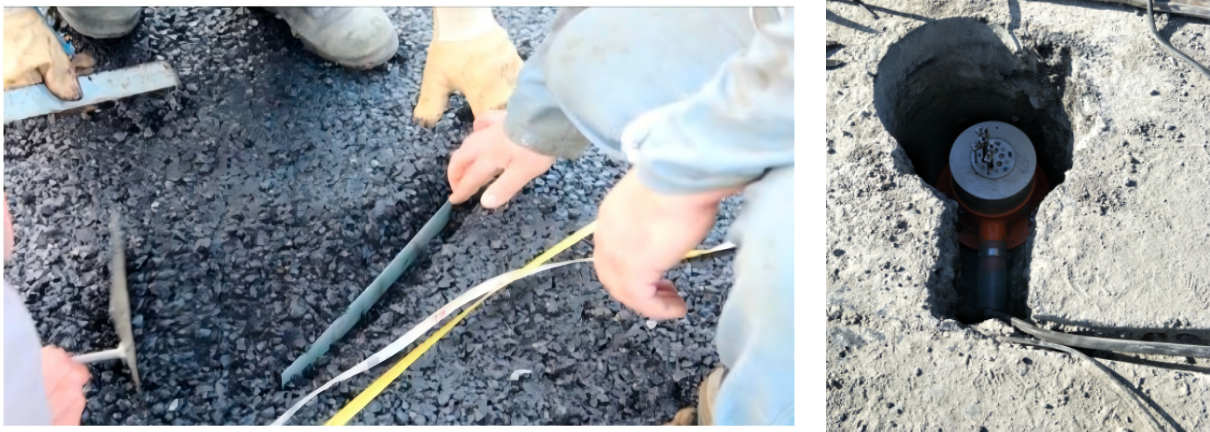
Figure 4. Sensors and equipment installation.
