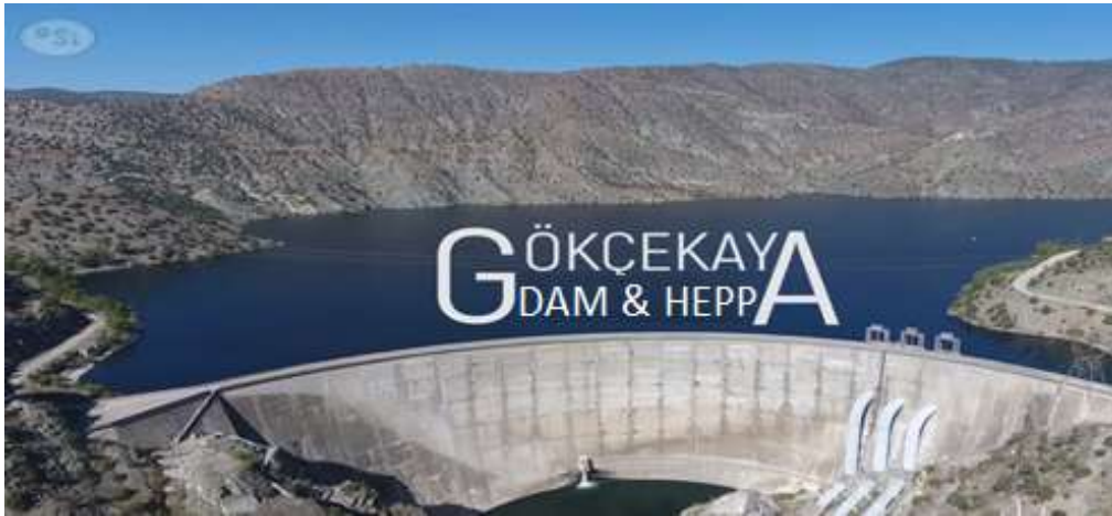
Figure 4. The existing hydro power plant demonstration [39]
