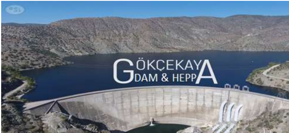
Figure 4. The existing hydro power plant demonstration [39]
