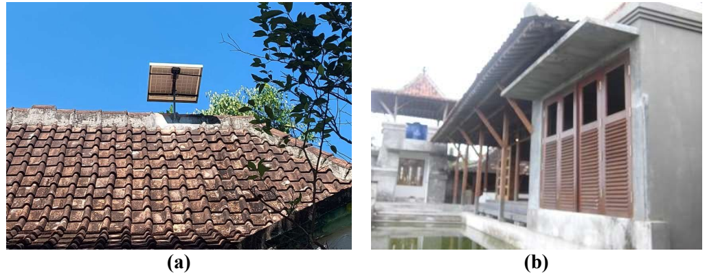
Figure 3. (a) Solar panels; (b) wide openings.
