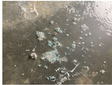
Figure 14. This is fireproofing on the floor that had sloughed off a column.
