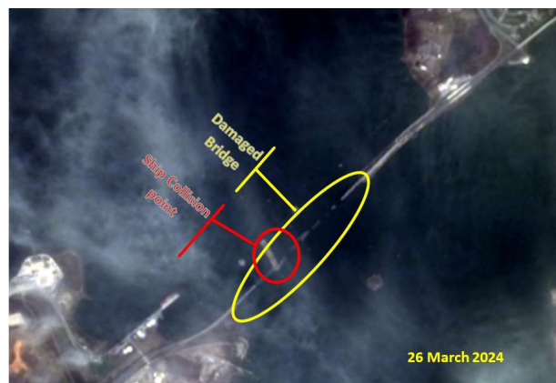
Figure 5. 26 March 2024—Post collision.
