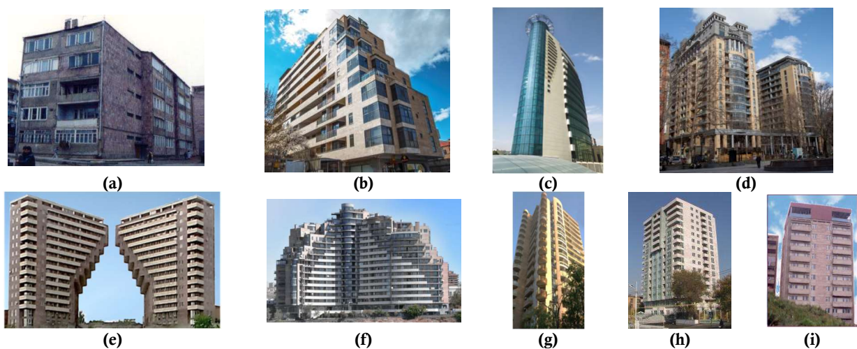
Figure 4. Some of the base or roof-isolated buildings are newly constructed or retrofitted in Armenia. (a) 5-story existing stone apartment building in Vanadzor retrofitted by base isolation for the first time in the world without interruption of the use of the building; (b) 11-story building of the multifunctional residential complex “Cascade”; (c) 20-story business center “Elite Plaza”; (d) 16- and 14-story buildings of the multifunctional residential complex “Arami”; (e) 18-story buildings of the multifunctional residential complex “Northern Ray”; (f) 16- and 13-story buildings of the multifunctional residential complex “Dzorap”; (g) 17-story building of the multifunctional residential complex “Baghramian”; (h) 17-story building of the multifunctional residential complex “Sevak”; (i) 9-story existing frame building protected by the roof isolation system—Additional Isolated Upper Floor—acting as a tuned mass damper.
