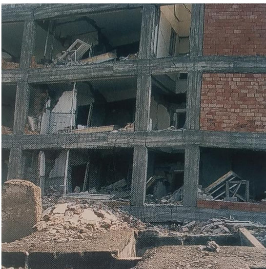
Figure 2. Damage and collapse of illiterately constructed non-load-bearing walls in frame buildings.
