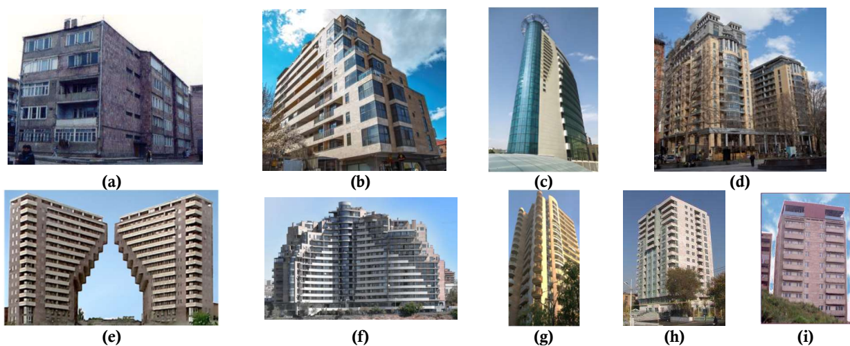
Figure 4. Some of the base or roof-isolated buildings are newly constructed or retrofitted in Armenia. (a) 5-story existing stone apartment building in Vanadzor retrofitted by base isolation for the first time in the world without interruption of the use of the building; (b) 11-story building of the multifunctional residential complex “Cascade”; (c) 20-story business center “Elite Plaza”; (d) 16- and 14-story buildings of the multifunctional residential complex “Arami”; (e) 18-story buildings of the multifunctional residential complex “Northern Ray”; (f) 16- and 13-story buildings of the multifunctional residential complex “Dzorap”; (g) 17-story building of the multifunctional residential complex “Baghramian”; (h) 17-story building of the multifunctional residential complex “Sevak”; (i) 9-story existing frame building protected by the roof isolation system—Additional Isolated Upper Floor—acting as a tuned mass damper.
