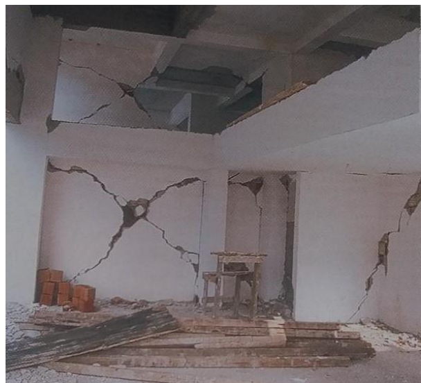
Figure 2. Damage and collapse of illiterately constructed non-load-bearing walls in frame buildings.
