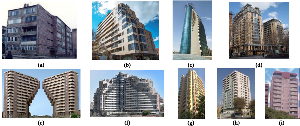
Figure 4. Some of the base or roof-isolated buildings are newly constructed or retrofitted in Armenia. (a) 5-story existing stone apartment building in Vanadzor retrofitted by base isolation for the first time in the world without interruption of the use of the building; (b) 11-story building of the multifunctional residential complex “Cascade”; (c) 20-story business center “Elite Plaza”; (d) 16- and 14-story buildings of the multifunctional residential complex “Arami”; (e) 18-story buildings of the multifunctional residential complex “Northern Ray”; (f) 16- and 13-story buildings of the multifunctional residential complex “Dzorap”; (g) 17-story building of the multifunctional residential complex “Baghramian”; (h) 17-story building of the multifunctional residential complex “Sevak”; (i) 9-story existing frame building protected by the roof isolation system—Additional Isolated Upper Floor—acting as a tuned mass damper.
