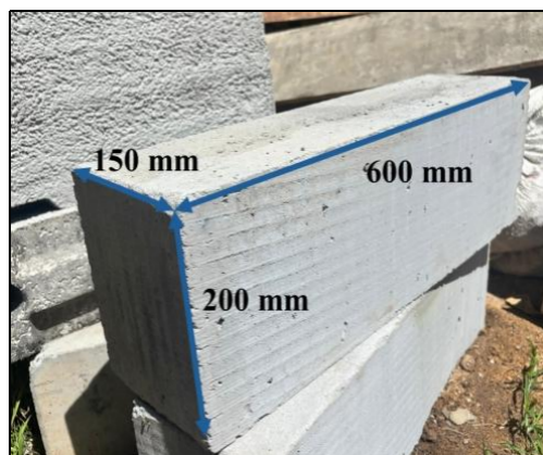
Figure 1. Alternative masonry: AAC block.
