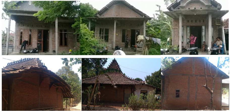
Figure 1. House in Demak (top) and house in Jepara (bottom).
