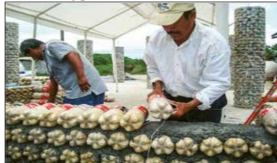
(d) Bottles laid and spaces filled with mortar.
