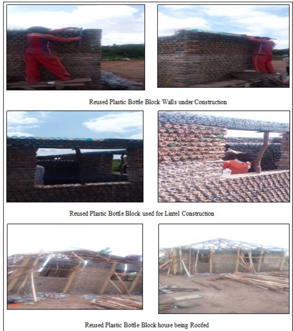
Figure 4. Plastic bottle house construction in Paipe village Abuja [36].
